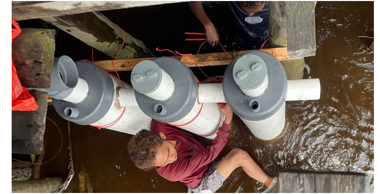
3 Installed the treatment tank on the house structure
