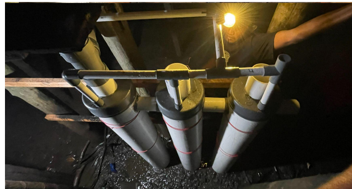
5 Installed the Tripikon ventilation system
