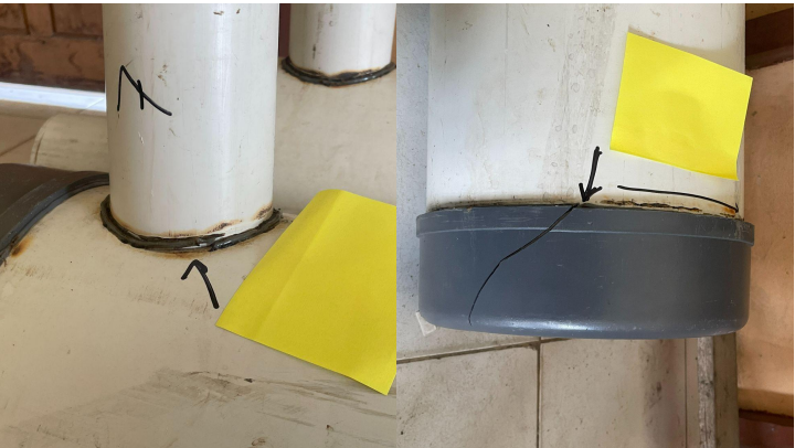
The connecting pipe between treatment tanks and 10-inch DOP, which was attached only with PVC welding, has come off and cracked.
