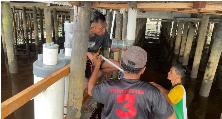
4 Connected the toilet outlet hole to Tripikon inlet pipe
