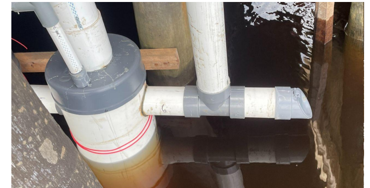
6 Installed the the Tripikon outlet pipes
