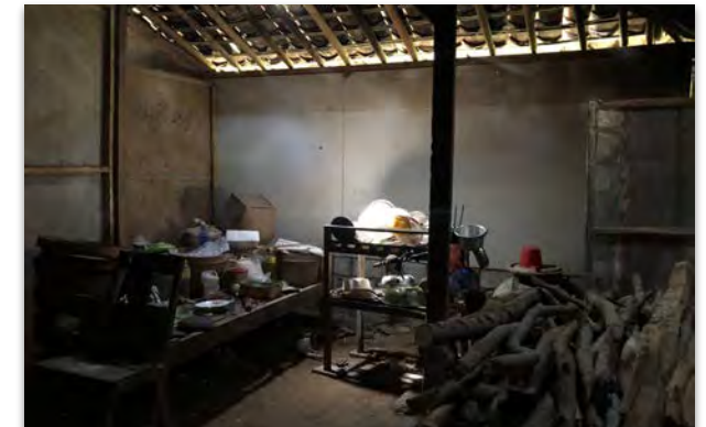
One of elder people's house is built with asbestos in the walls and has a dirt floor.
